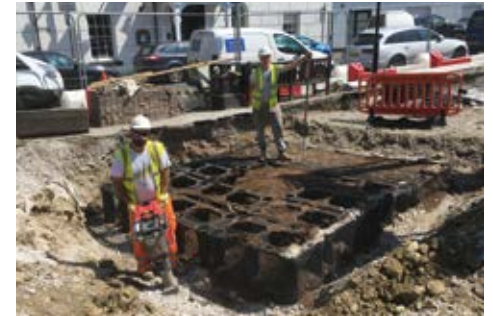
Excavation of the tree pits
